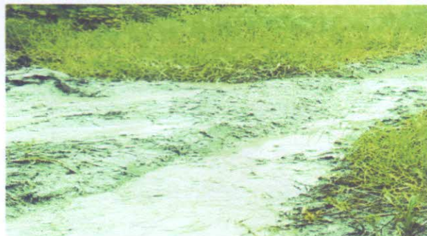
BACK FILLING OF THE REPAIRED POINT
