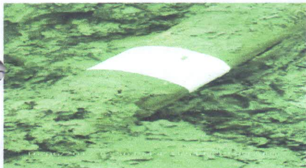
REPAIR WORK DONE BY NAOC REPAIR TEAM
